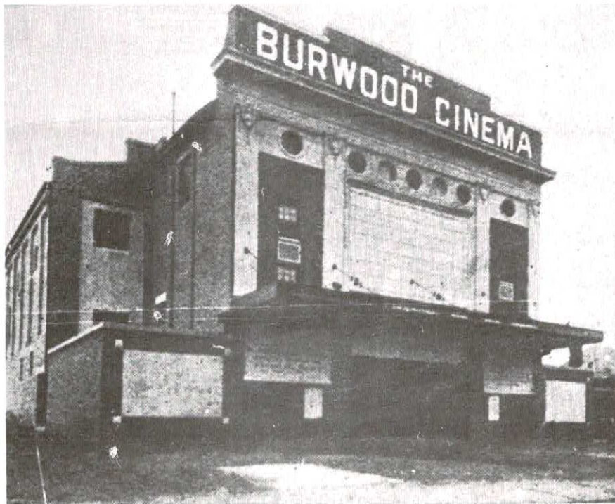
Exterior of the new Theatre at Burwood.
