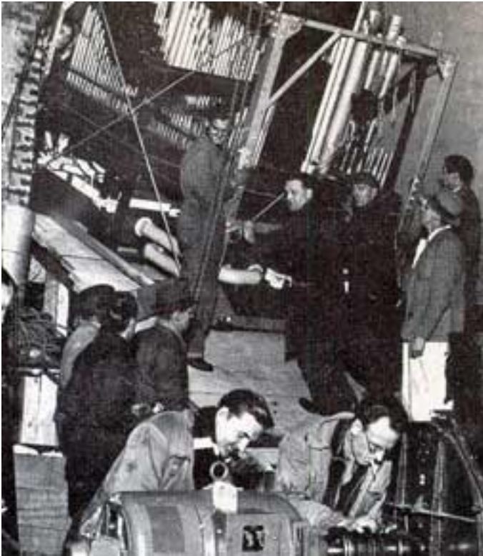
One section of the organ being moved into one of the many theatres. The motor in the foreground was one of several, due to the varying electrical currents.
