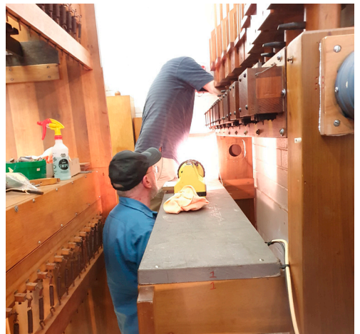
The trunking to the 16' Tibia offset chest back in place following reinstallation of the refurbished chest
