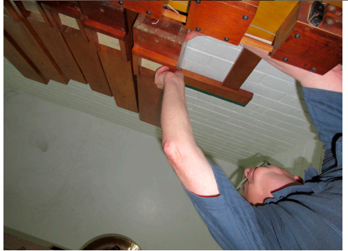
John Parker above & John Weismantel below replace the 8' tibia offset pipes after restoration of the chest
