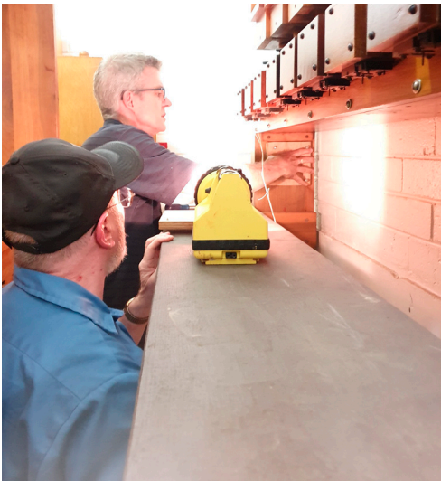
The trunking to the 16' Tibia offset chest back in place following reinstallation of the refurbished chest
