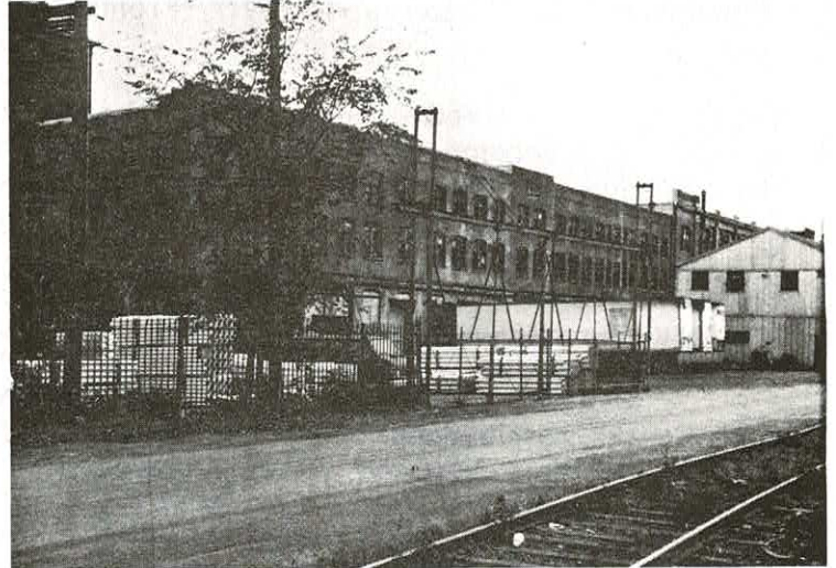
Rear of the factory, showing loading dock area. Railroad spur over which organs were shipped, is shown.
