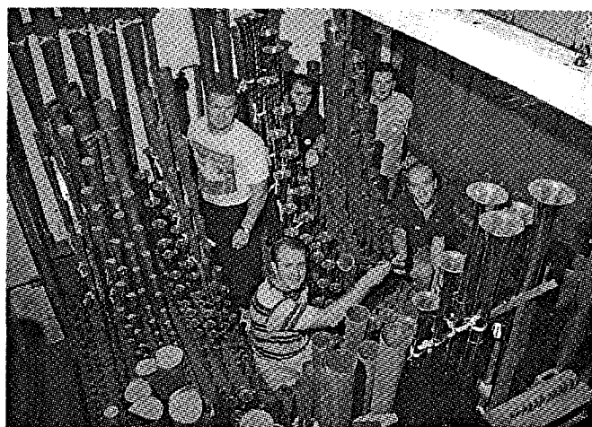
19th August, 1997 - the first pipe is removed from the Solo Chamber
