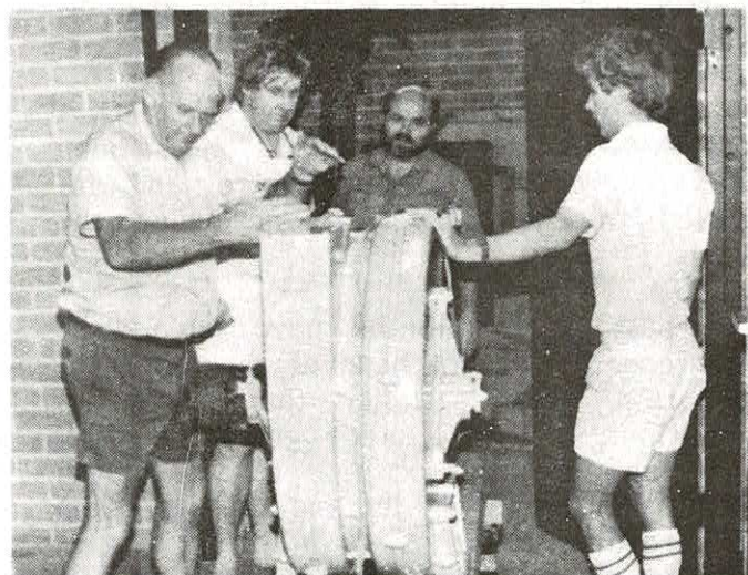
The blower unit, mounted on temporary castors, being wheeled into position.
