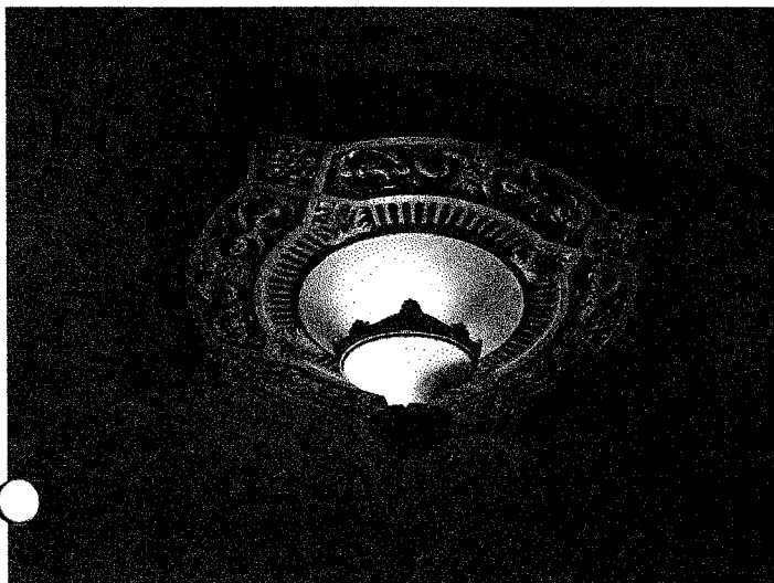
Plaster roof light fitting
