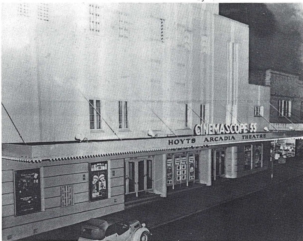
EXTERIOR OF THE ARCADIA IN 1956
